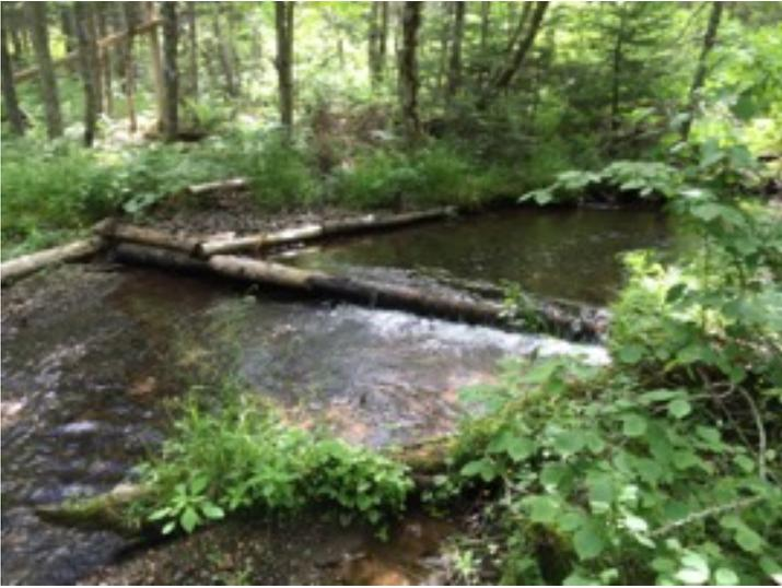
A digger Log before repair. Water should flow over not through.
